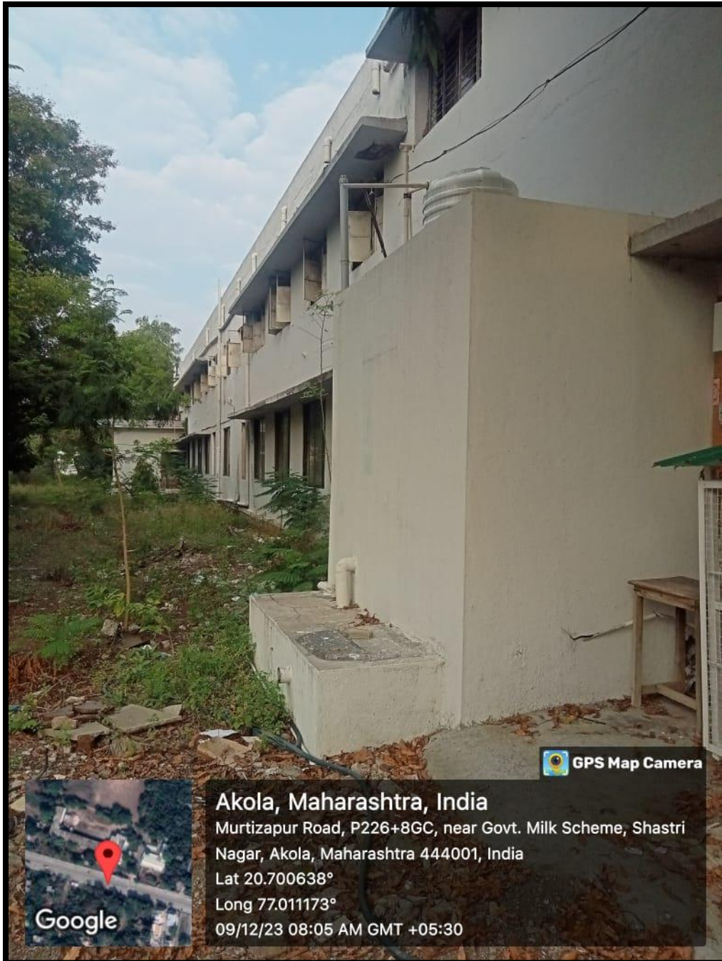
Liquid Waste management – Drainage facility
